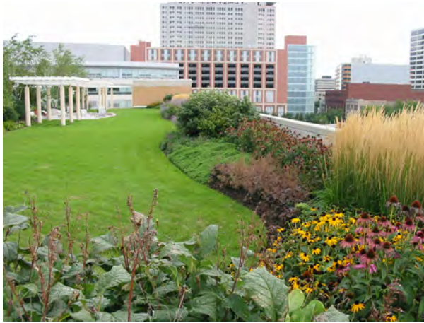
Figure 16: Intensive green roof
